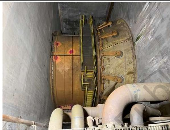
Photo 38: Bulb turbine distributor
