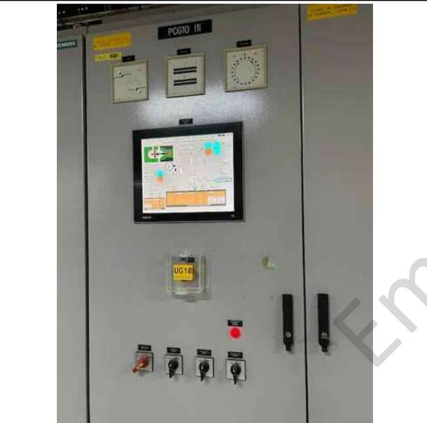
Photo 40: Redundant operations example (local controls for generating unit 10)
