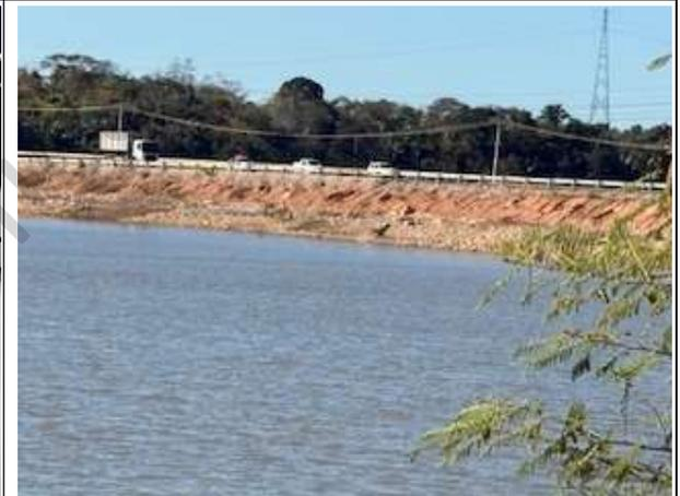
Photo 3: BR-364 highway raised by SAE after the 2014 flood and the increase in the reservoir operating level to 71.3 masl
