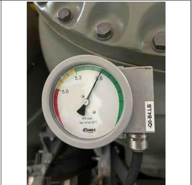
Photo 42: SF6 used in electrical equipment
