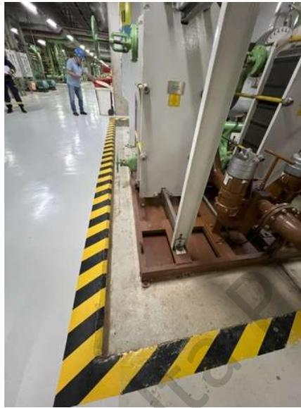
Photo 50: Oil spillage containment basin
