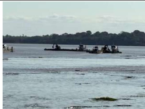
Photo 19: Logboom and macrophyte cleaning operation near the dam
