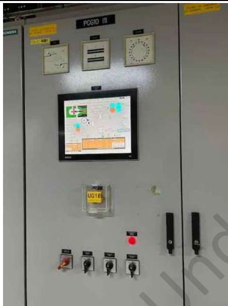
Photo 40: Redundant operations example (local controls for generating unit 10)
