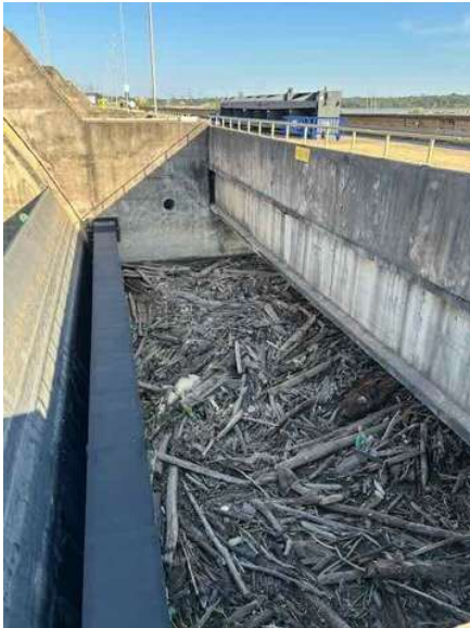
Photo 22: Debris including logs, trash and dead animals collecting at main spillway
