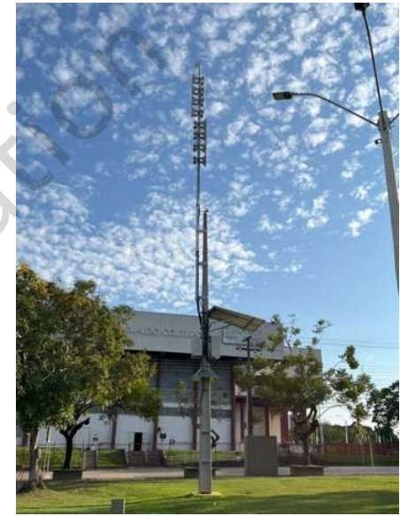
Photo 129: Flood warning siren in Porto Velho, provided by SAE
