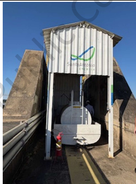
Photo 71: Equipment for emergency operation of spillway gates
