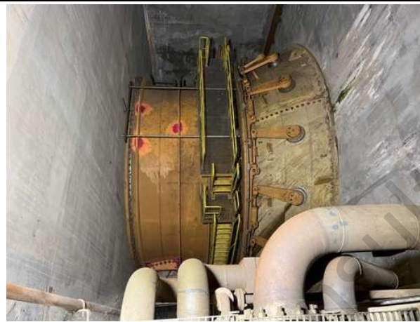
Photo 38: Bulb turbine distributor
