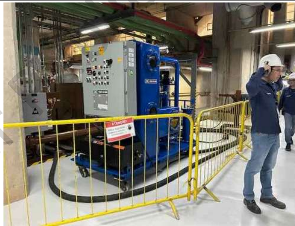
Photo 53: Safety barriers, PPE, oil containment
