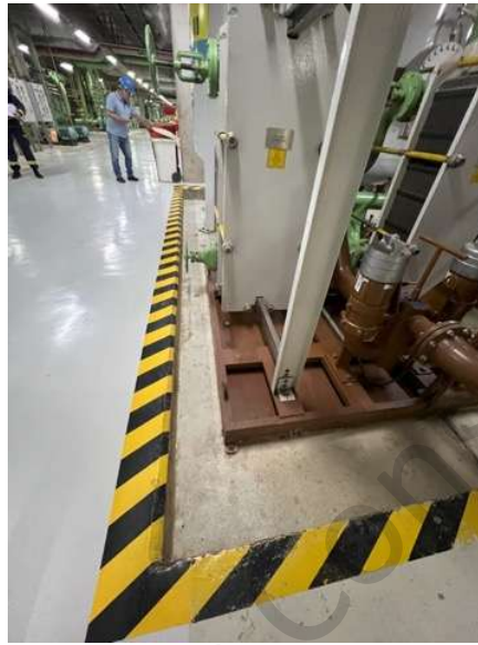
Photo 50: Oil spillage containment basin
