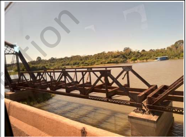
Photo 111: Madeira-Mamoré railroad bridge, on raised foundations
